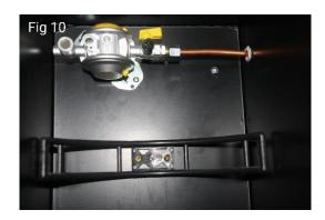
Try to avoid a sloping downward connection from cylinder to regulator, as the regulator may become clogged and blocked with residue from the cylinder.
