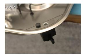
For connection of the hob to a suitable regulator, 8mm Copper pipe is fitted from the steel stem underneath the hob and run to the regulator's pre-determined position. A compression joint such as seen in 34 is used to connect the 8mm pipe to the steel stem of the hob.
