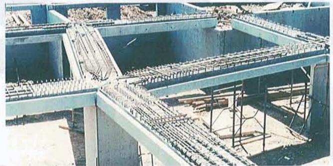
Unusual or complicated details are achievable with precast components.
