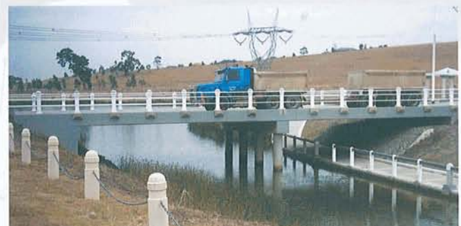
Hollow Core planks are used for the economic construction of bridges.
