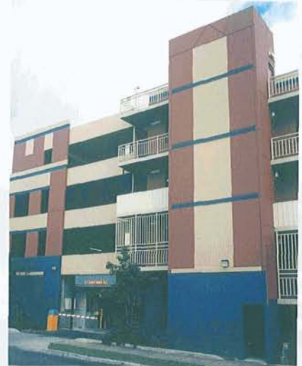
Top: This multi storey car park development constructed using Hollow Core planks supported on a steel frame structure.
