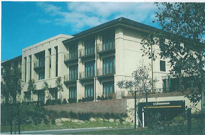
Top: This multi storey car park development constructed using Hollow Core planks supported on a steel frame structure.
