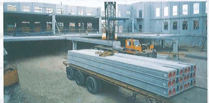
Hollow Core planks, along with precast columns, beams and panels provide open unpropped floors resulting in significant construction time savings.
