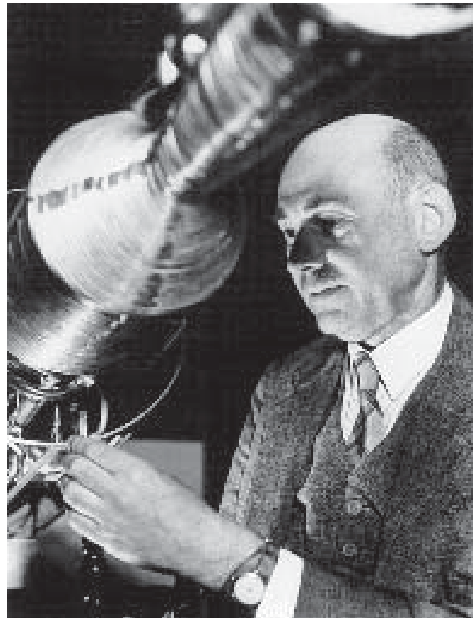
Dr. Robert H. Goddard makes adjustments on the upper end of a rocket combustion chamber in this 1940 picture taken in Roswell, New Mexico.
