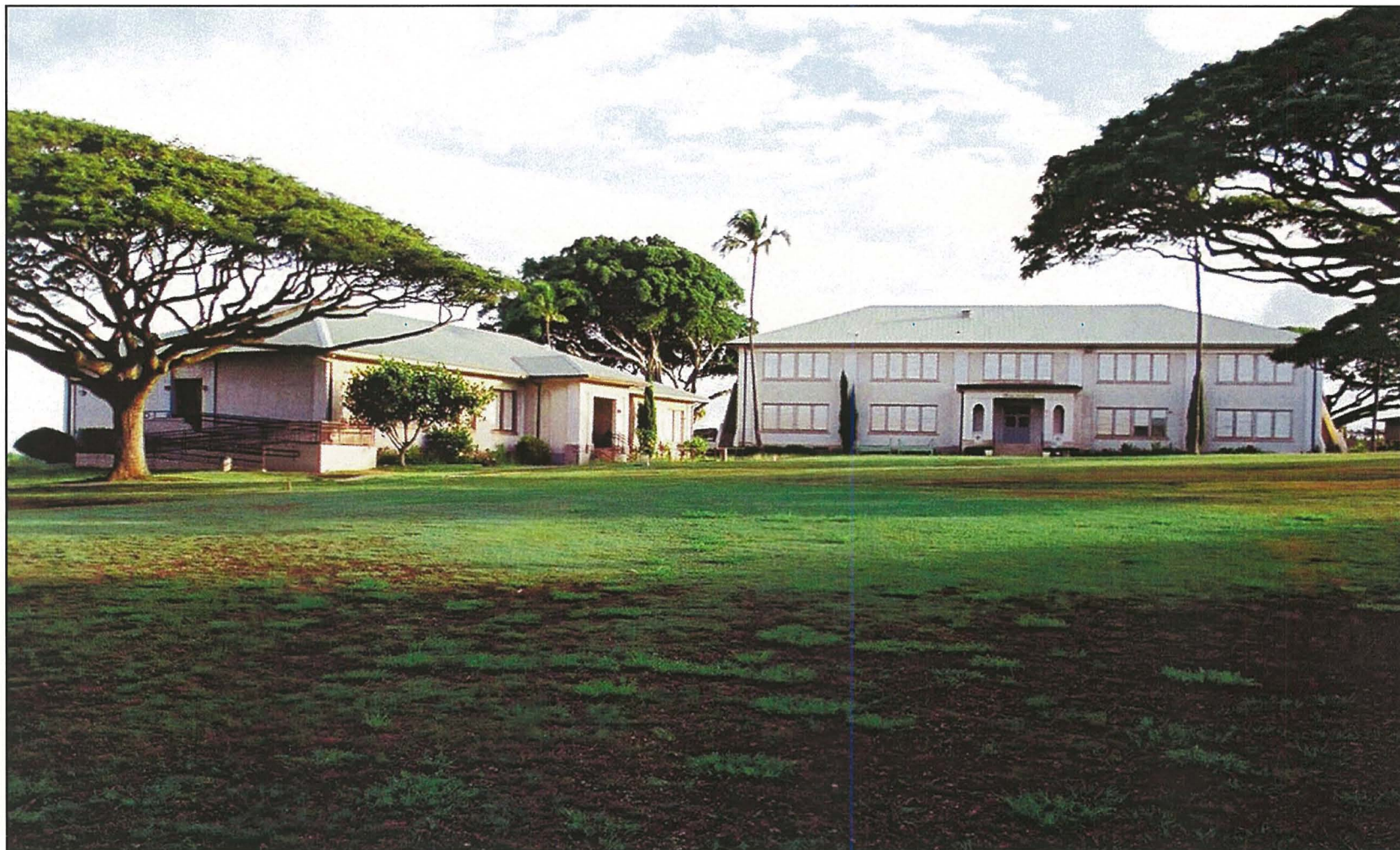
Figure 8. Present-day classroom and administrative office structures at the Pā'ia Elementary School. “Building B,” originally constructed between 1930-1936, is shown on the left and “Building A,” constructed in 1926, is shown on the right. (Building designations are taken from the 1992 Federal Register Nomination Form).
