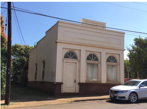
Figure 49: Example of 1913 commercial building, Paia, Maui
