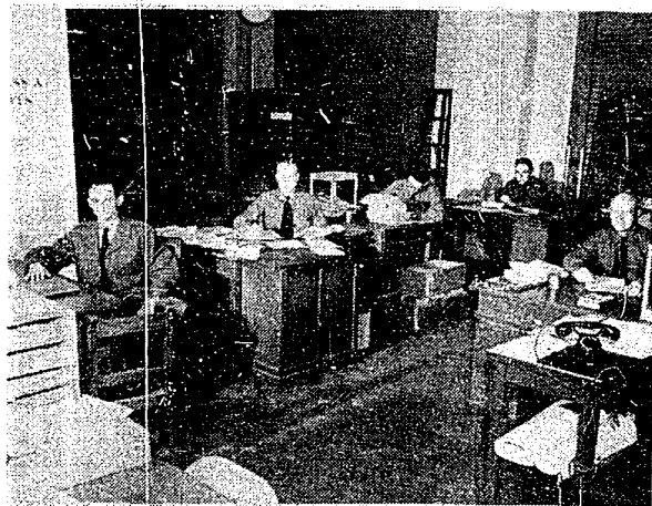
Technical Department Offices (Meiji Building)
