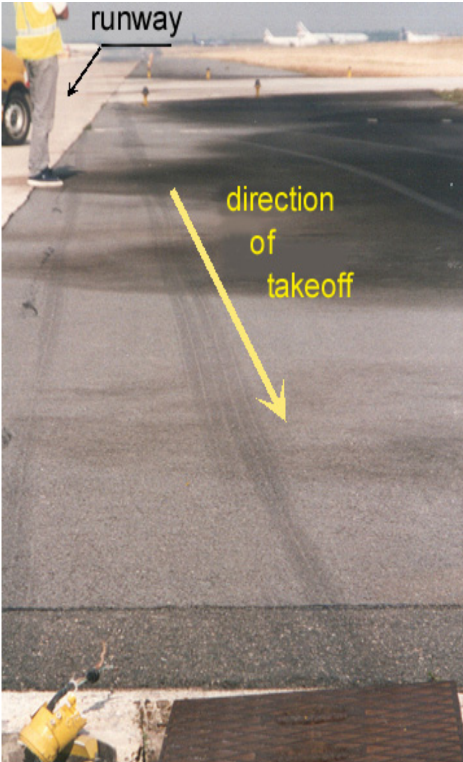
Figure 25: Marks of left bogie tyres and edge light
