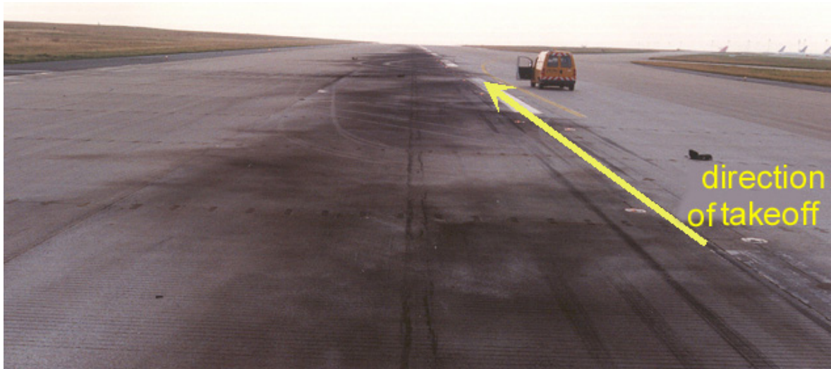
Figure 26: Soot marks on the runway
