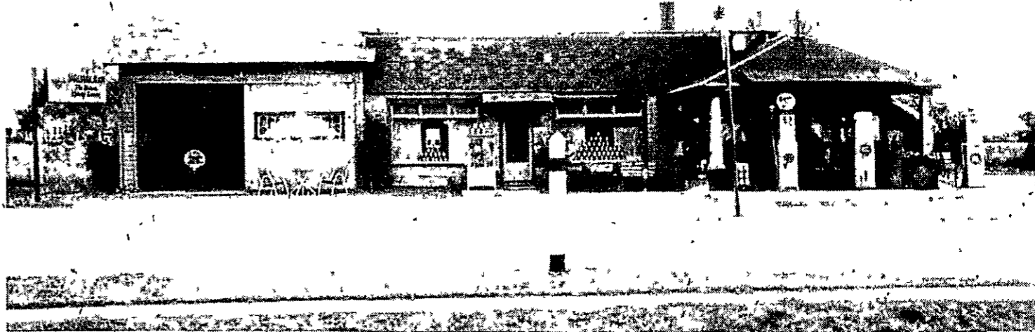
OLD SERVICE STATION HAS A ROLE
