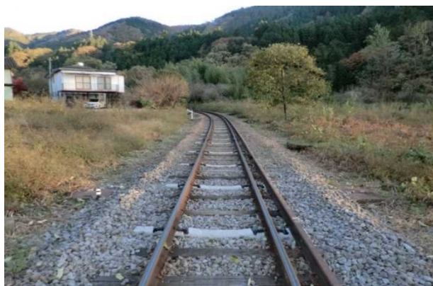
Figure 8: Example of partial replacement with PC sleepers
