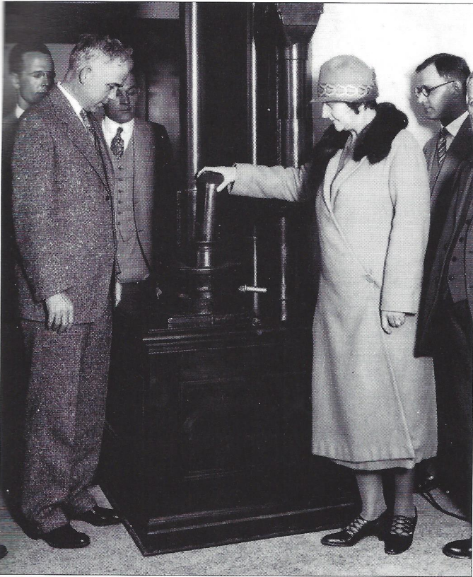
Mellie Esperson shows off the pneumatic tubes in the new Neils Esperson building to Mayor Oscar Holcombe and other dignitaries. Holcombe is left front, looking down. The tubes conveyed messages between the Esperson building and the Harris County Courthouse a half-mile away. Courtesy Houston Metropolitan Research Center, Houston Public Library.
