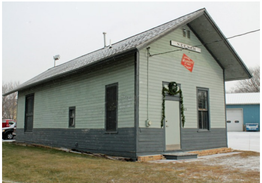
The home of the Neenah Model Railroad Club is the depot built by the Milwaukee & Northern Railroad in Neenah, Wisconsin during the 1870's. Photo by Dave Nitsch
