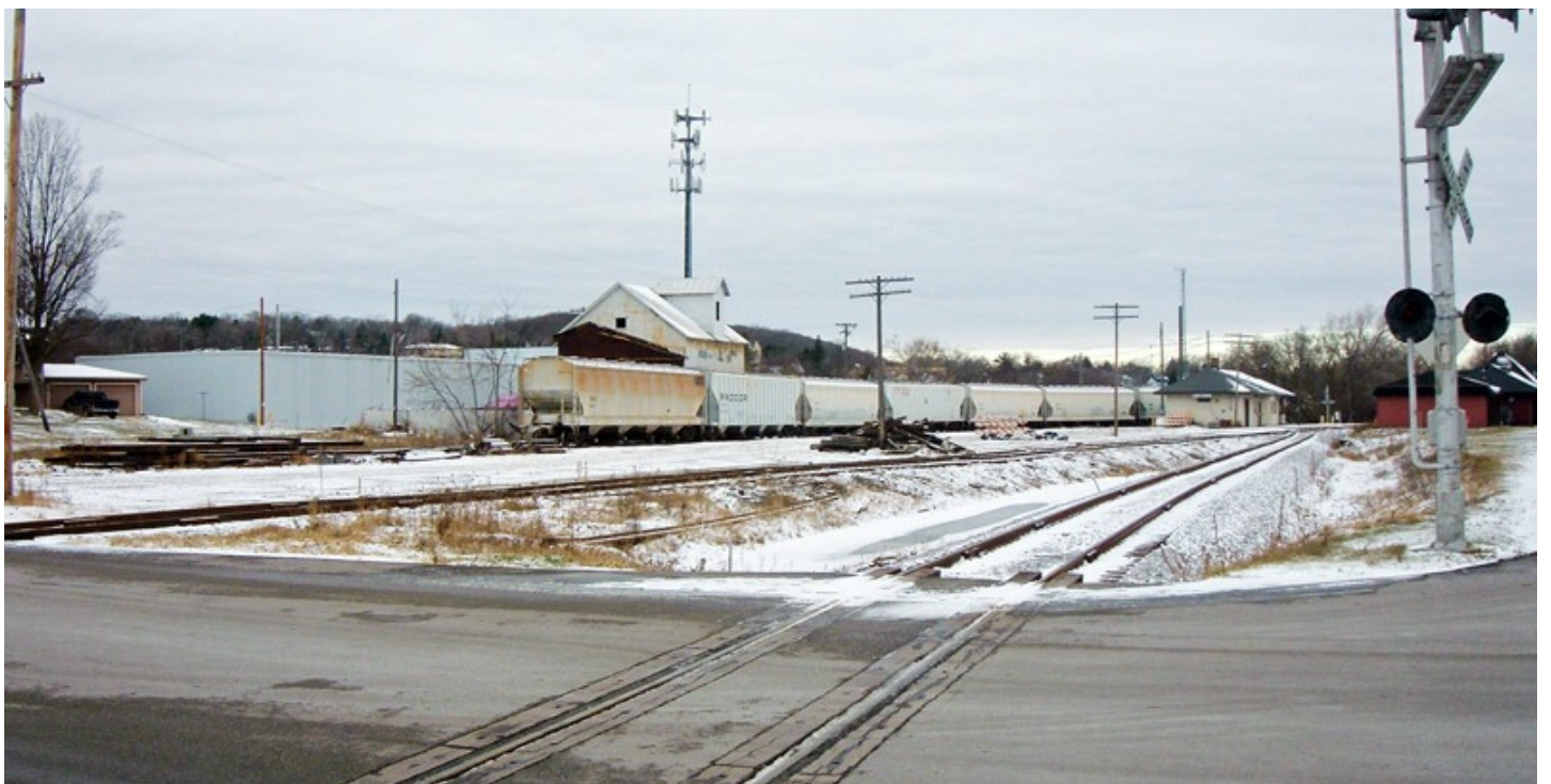
We are back in Plymouth again, looking north. The covered hopper cars are full of plastic pellets that get loaded into trucks and hauled to nearby plastic molding places. The cars are sitting on the old Milwaukee Road team track. There was a railroad freight house and a private warehouse on the track at one time. Today, the trucks pull up alongside the cars to unload them. The railroad also uses the site as a staging area for their maintenance. The tan depot is the old Milwaukee Road depot, and the red building behind the crossing signal is the old Chicago & Northwestern depot. The track in the foreground is the old C&NW line from Sheboygan to Fond Du Lac. The tracks crossed over each other just past the depot, and continued on next to each other for a few miles before separating. The Milwaukee depot is used by the railroad, and the C&NW depot is a restaurant. The site is approximately the same as it has been for 100 years. The difference is in the details. If you are modeling the modern era, do it as the photo shows. Don't forget to add the abandoned tracks in the weeds and
