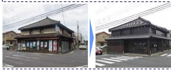
The dislocated tiles on the heavily damaged rooftop were placed back in position and plasters peeling off from the walls on the second floor and below the eaves were repaired.
