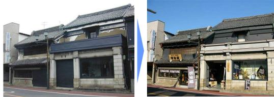
The façade of a Kurazukuri-style building using steel sheet was restored to its original look and the walls were repaired with black plaster.
