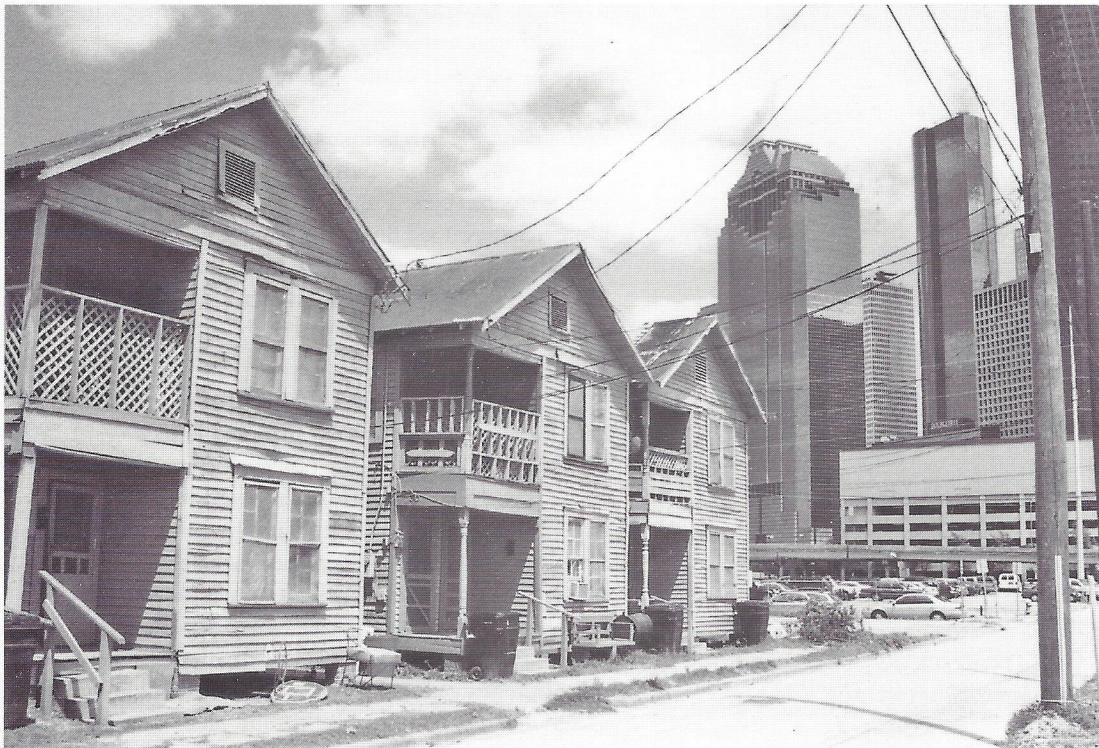
Now in the shadow of downtown Houston's towering skyscrapers, much of the Freedmen's Town neighborhood (left) is falling victim to gentrification. Inner loop real estate is becoming popular once again and developers are taking advantage of this change in attitude. Older homes throughout the Fourth Ward and other neighborhoods such as Montrose are being torn down as fast as new luxury town homes are erected.
