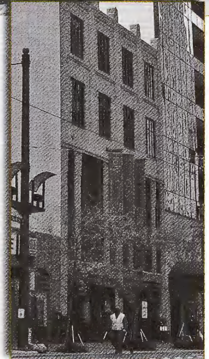
In 2002, the Holy Cross Chapel restored the façade to its original appearance, and later received a Good Brick Award from the GHPA for their efforts.
