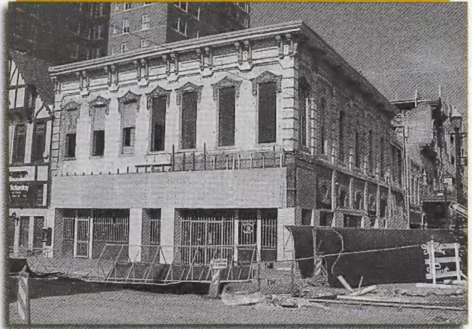
The slipcovering of 1879 Stegeman Building at 502 Main did not fully obscure the upper ornamental brackets and cornice capping the building. These visible remnants of the past helped to inspire the building tenant to remove the slipcover and begin restoration work on the original façade beneath.
