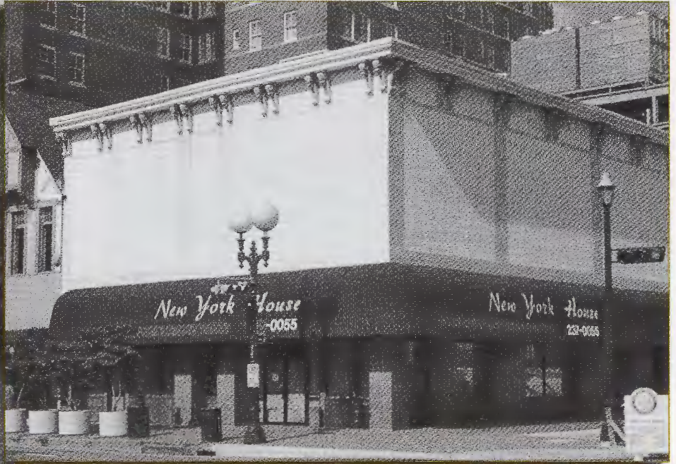
The slipcovering of 1879 Stegeman Building at 502 Main did not fully obscure the upper ornamental brackets and cornice capping the building. These visible remnants of the past helped to inspire the building tenant to remove the slipcover and begin restoration work on the original façade beneath.
