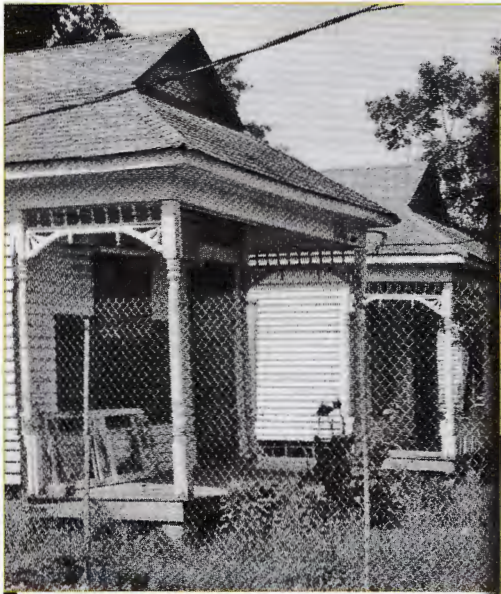
Saved from demolition and donated to the Greater Houston Preservation Alliance by the Cannata family, the late-nineteenth century Victorian "Cannata Houses" on Decatur Street in the Old Sixth Ward Historic District were renovated, restored, and sold as affordable housing in cooperation with the City of Houston's HOME Program and the Old Sixth Ward Community Development Corporation (now Avenue CDC). The after photo was taken in 1995 as GHPA volunteers were setting up for the dedication ceremony.
