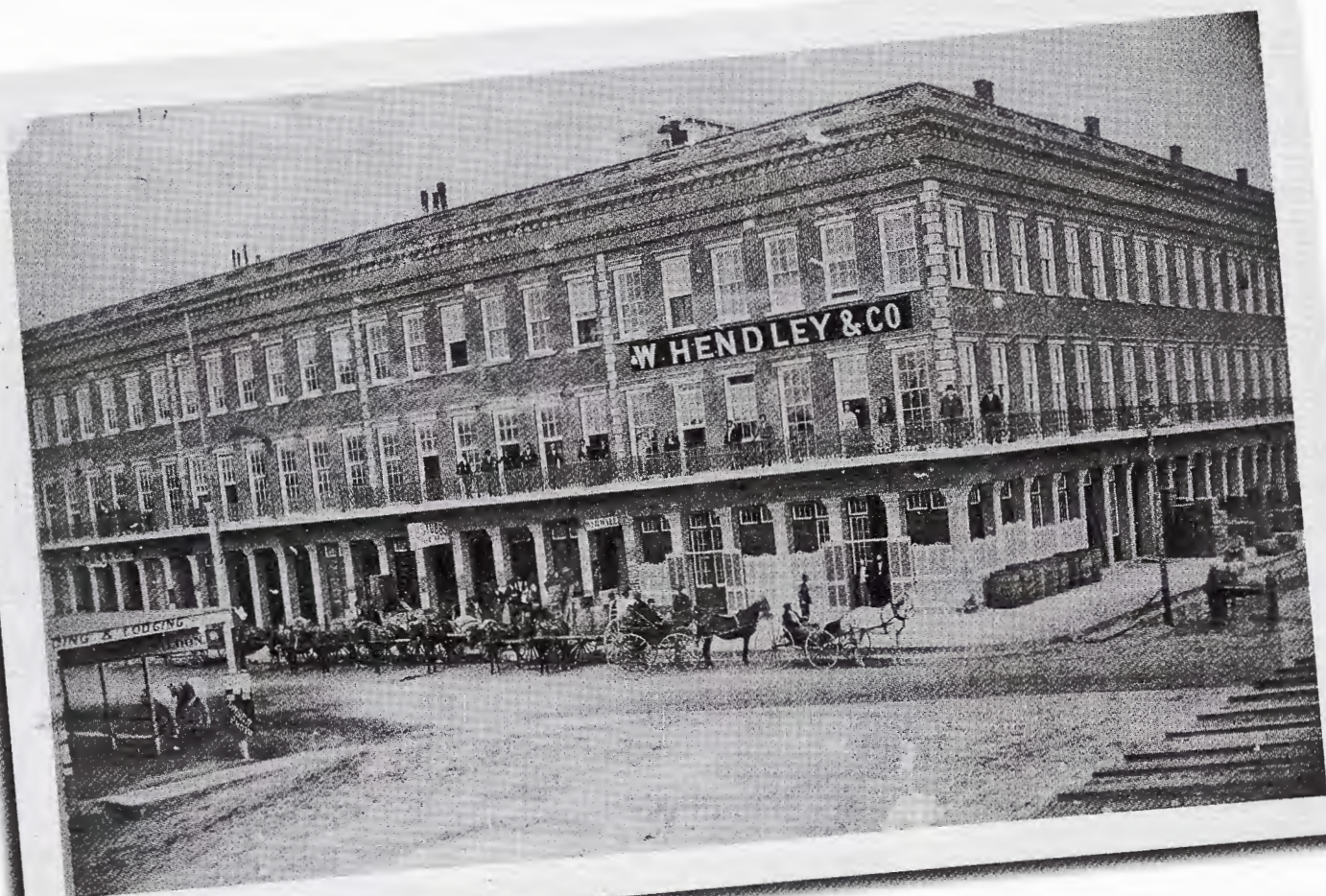
The 1858 Hendley Building, Galveston's oldest brick and granite commercial building, is on Galveston Historical Foundation's "Heritage at Risk List." Historic preservation graduate students from Ball State University's College of Architecture and Planning completed a week-long survey of the building in March 2005. This resulted in a full report on the status of the structure, including options for rehabilitation and future use. These options will be explored further.
