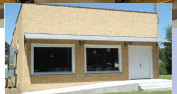
Renovations at a former grocery store, located on Hwy. 77, are now complete and the building is ready for use as Rosedale's Community Center.
