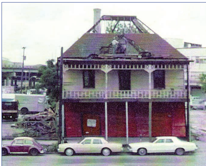
The Cadillac Bar under demolition in 1971. The Cadillac Bar converted an old house into a commercial property on the Stockbridge Ford land near the location of Samuel Stockbridge's home. The building was made of heart cypress or pine planks that were two stories in length. The building was all board and batten construction, solid as a rock, and probably built sometime in the 1840s or early 1850s.
