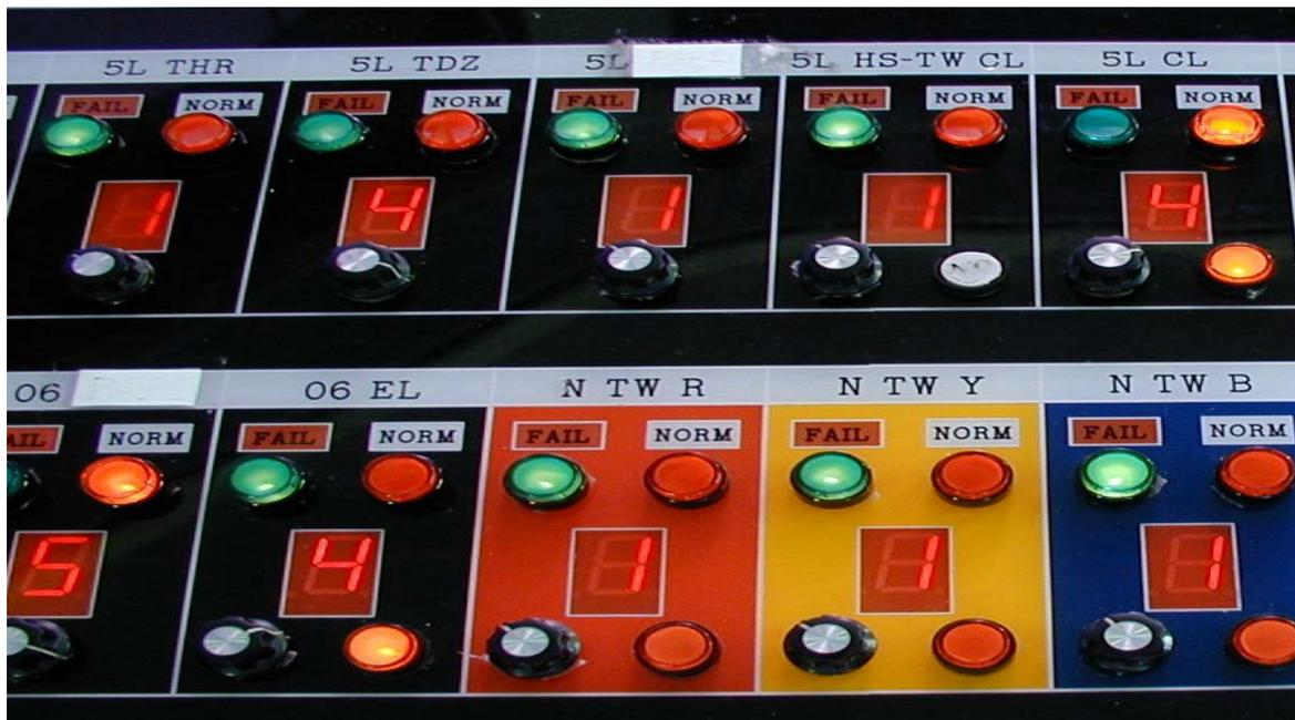
**Figure 1.10-13 Airfield lighting control panel in the control tower**
