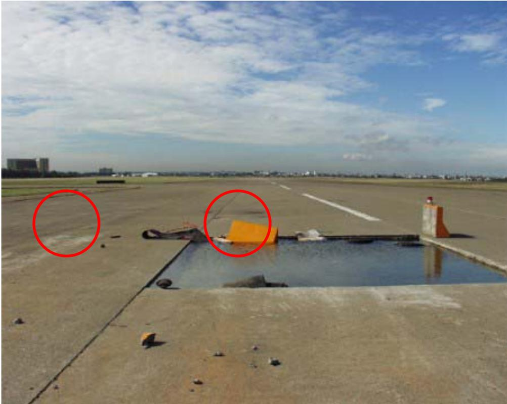
Figure 1.12-3 Initial impact point (shown circled)
