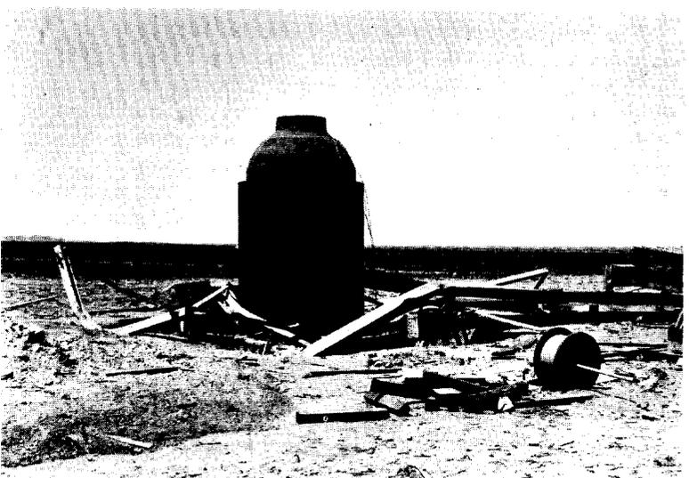
Damage to the instrument shelter at North 1000 is shown in the two top photos. At the bottom, Jumbo stands unscathed, its tower crumpled around it.
