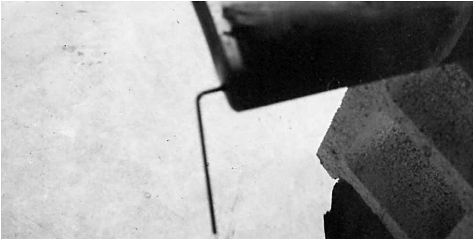
Through-bolt is secured using allen wrench through recoil pad.
