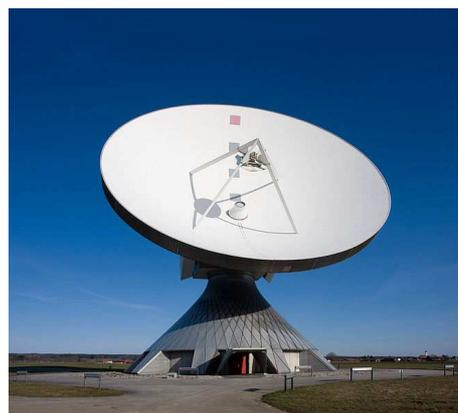
A plane wave has the same phase at  $D$  and  $B$ . Using Snell's law and some calculus you can then show that the shape of the dish must be a parabola for the reflected waves all to be in phase when they reach a single point (the focal point). There is a nice simulation of this in Ripple.
