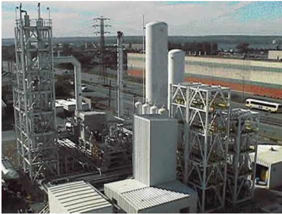
Figure 2.7. Atomic Energy of Canada Ltd. advanced heavy water pilot plant, Hamilton, ON. Photo courtesy Atomic Energy of Canada Ltd. This plant produced about 1 ton of heavy water per year. A scaled up version of it would be more efficient and cleaner than the old Bruce Point plant, shown above.
