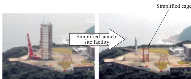
Fig. 11 Mobile launch pad with a compact cage
