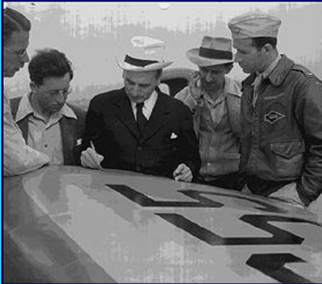
First composite **castable** solid rocket propellant by J. Parsons at GALCIT:  $KClO_4$  + asphalt, June 1942, JATO
