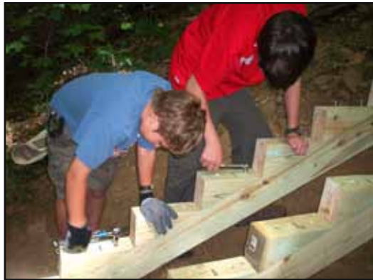
Shawn Bishop (on the left) and Mike Swann, assembling the frame for Brian Niebanck's steps —Photo by Ross Lanius
