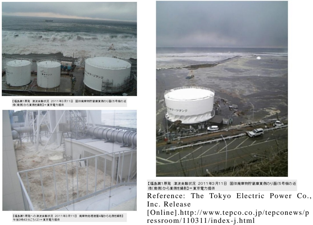
Fig. III-2-4(b) Photos showing plant damages at the Fukushima Dai-ichi NPS.
