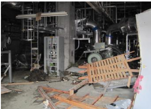
Damages of reactor building and emergency diesel generator (Unit 1)
