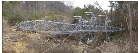
Collapsed tower
