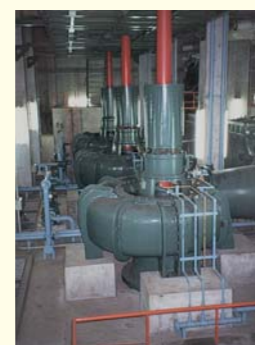
⑤給水所 (本郷給水所配水ポンプ) Water Supplying Station (Hongo Water Supplying Station Distribution Pumps)
