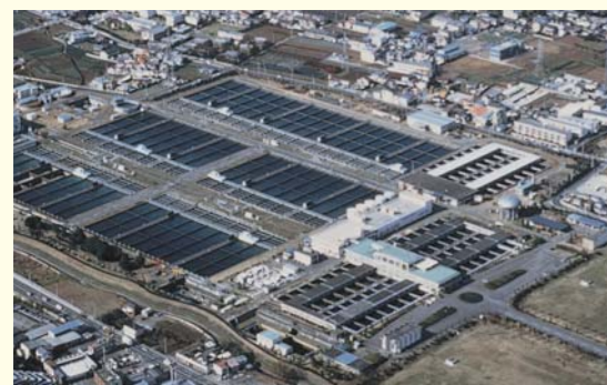
④浄水場 (東村山浄水場) Purification Plant (Higashimurayama Purification Plant)
